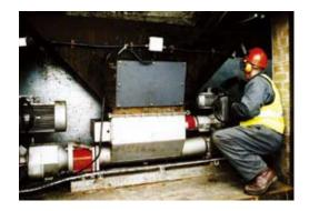
A W064 model installed at a sewage treatment works to control sewage odours, caused by a belt press feeding dewatered sludge cake directly onto an open-air conveyor and into an open skip for disposal. The cast iron W064, with an integral bridge breaker fitted as an option, delivers the sludge cake at the required rate of 2.5m3/h and pressures of up to 12 bar. It operates eight hours per day, six days a week and daily fills up the four enclosed skips with sludge cake.
