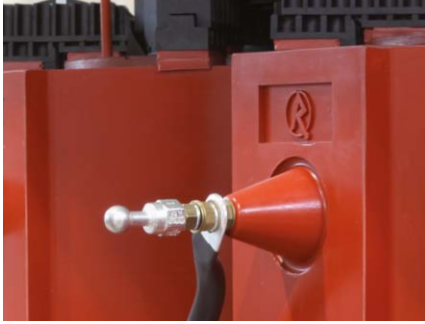
HV winding connections with ball connection bolts
