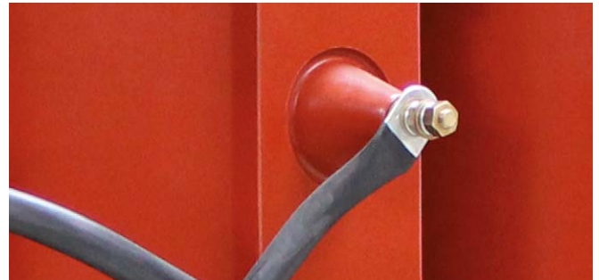
HV winding connections
