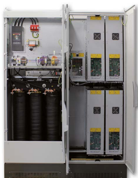
EOS System 800 kW ± 20 %
