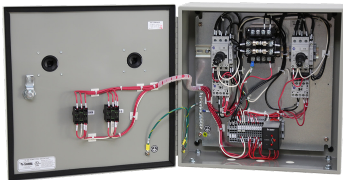
Inside view of control panel
