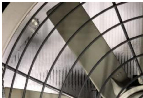
Ice built-up might occur on the air outlet side – but it depends on the evaporator design. Here the pipes closest to the expansion valve are on the air outlet side
