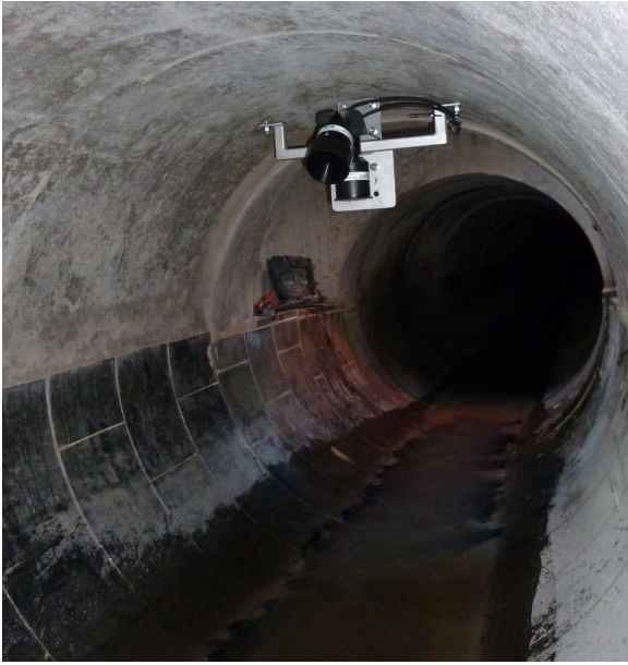
MicroFlow-i Measuring Flow Velocity
