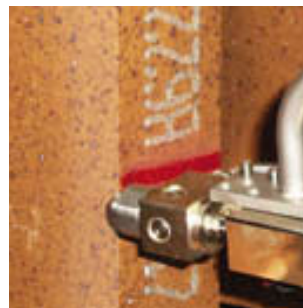
Chimney stone line-marking for correct installation
